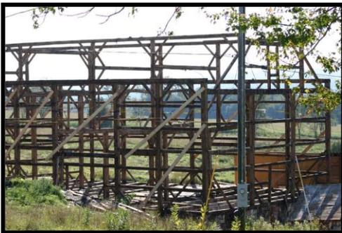
nearly complete. Beams going cross-ways measure 44 feet and length-ways up to 56 feet. The post and beam
